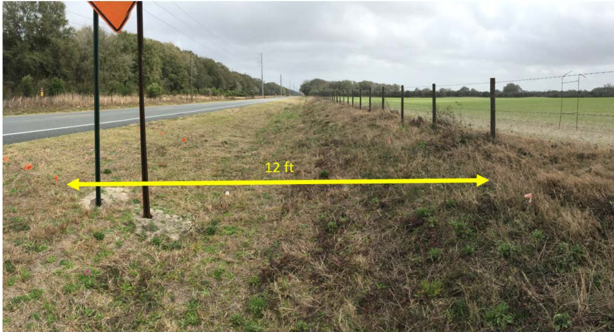
Figure 35. Linear ditch construction site
