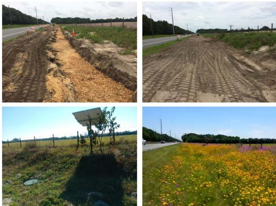
Figure 38. Construction and operation strategy in the field (upper left: construction phase; upper right: completion of construction of B&G media section; lower left: operation of pumps with solar panel in the middle of B&G media and woodchip sections; lower right: operational phase of B&G media and woodchip sections)
